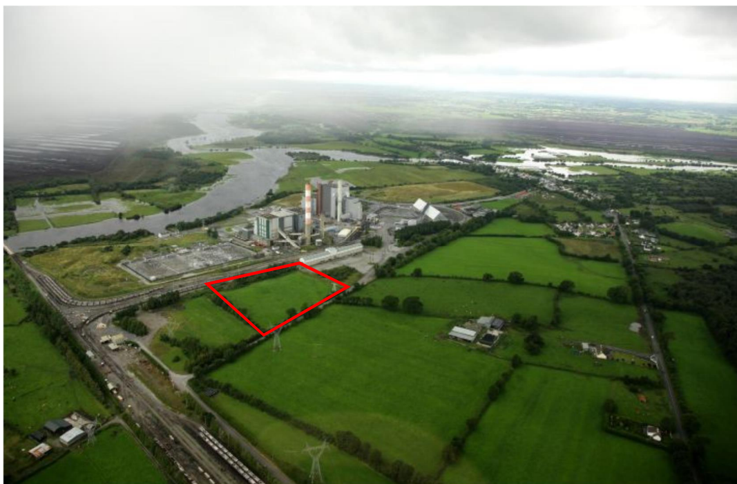
Figure 3 OPW Flood Record Photo (August 2008)
